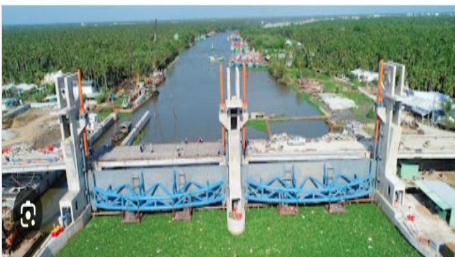
Sluice gate for used irrigation system
